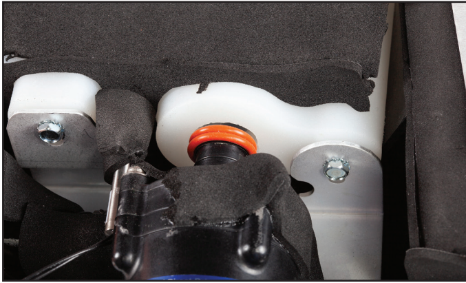
Fig 8-60 Install Chiller Pump with O-Rings on Pump Outlet
